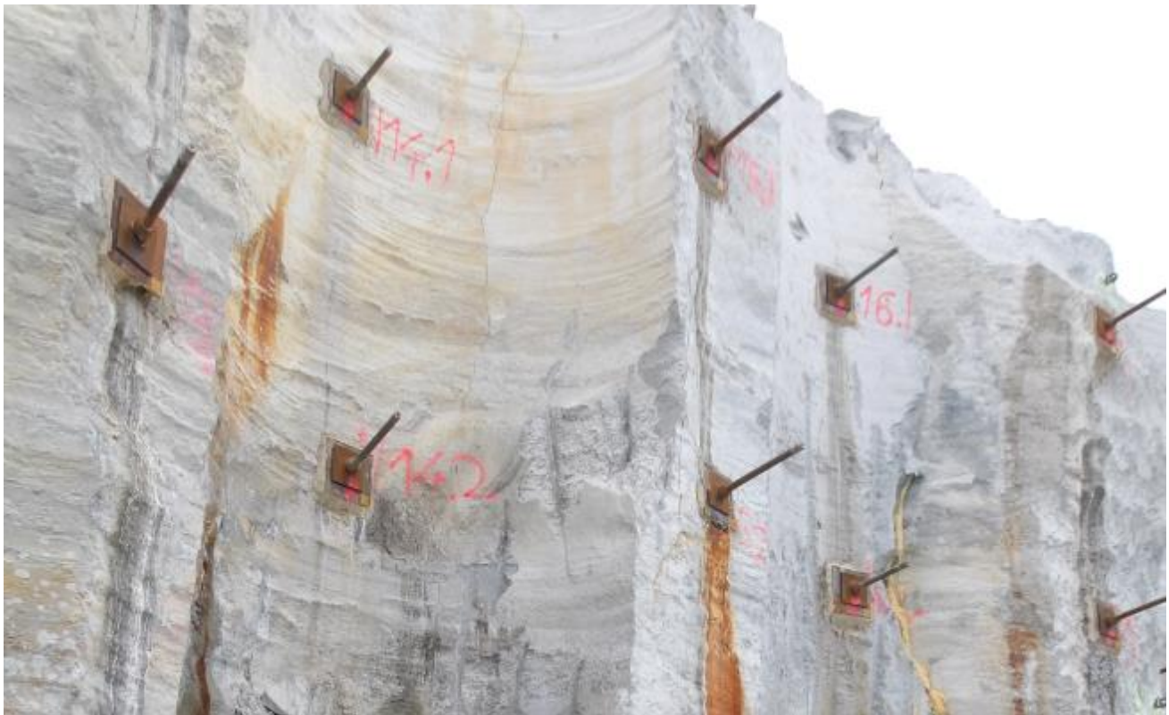
The construction site of the Paks II Nuclear Power Plant, nuclear island of Unit 5 the location of the lower part of the Northern working pit reinforced with soil nails (The photo was taken by HAEA.)
